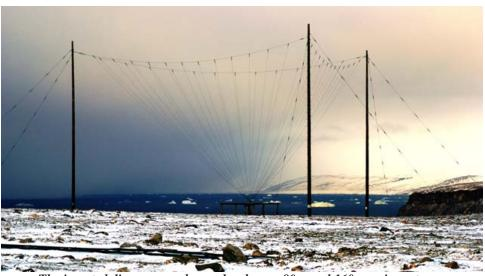
The inverted discones can be used as low as 80m and 160m, using a tuner.
