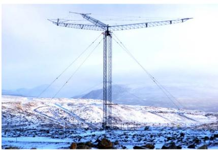
The log periodic was finally fixed. The feedline was crushed by snow removal equipment. Even so, the rotor is not working and it only faces in one direction.
