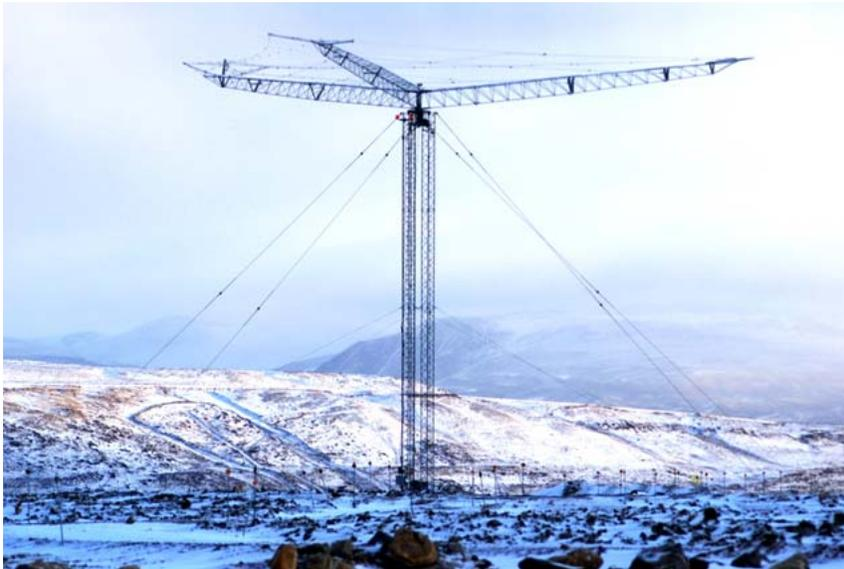
*The log periodic was finally fixed. The feedline was crushed by snow removal equipment. Even so, the rotor is not working and it only faces in one direction.*
